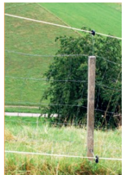
Figure 10: Electrified mesh wire
