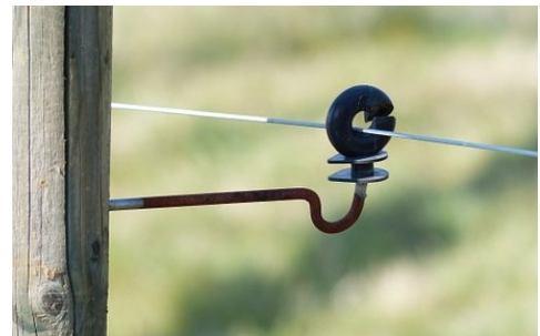
Figure 9: Electric wire running outside the fence
